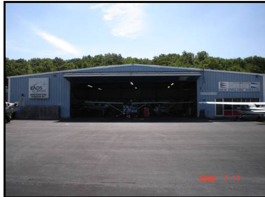
New England Aviation Hangar
